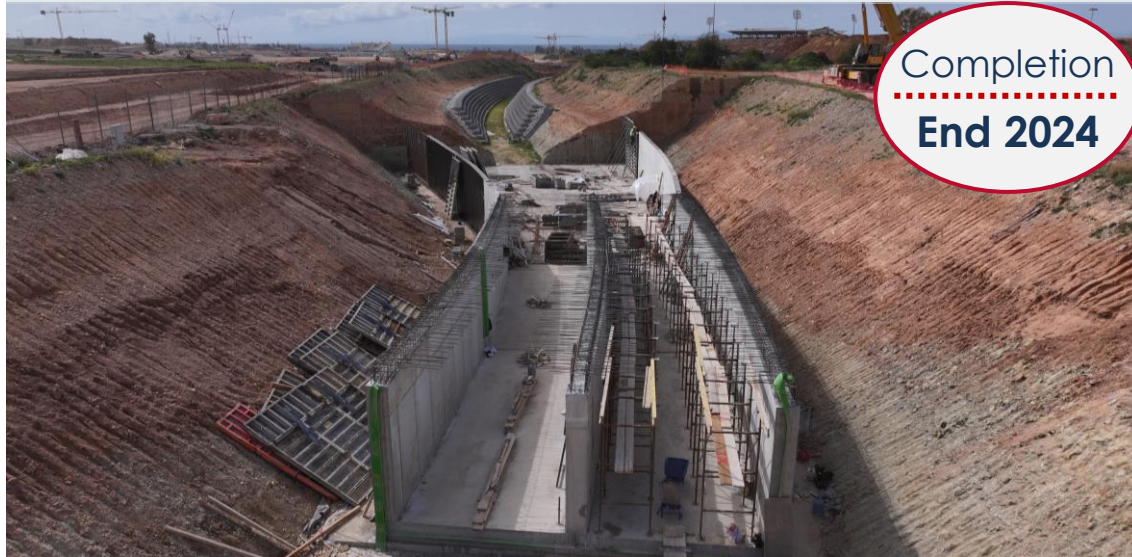
Trachones Stream 80% of excavations
