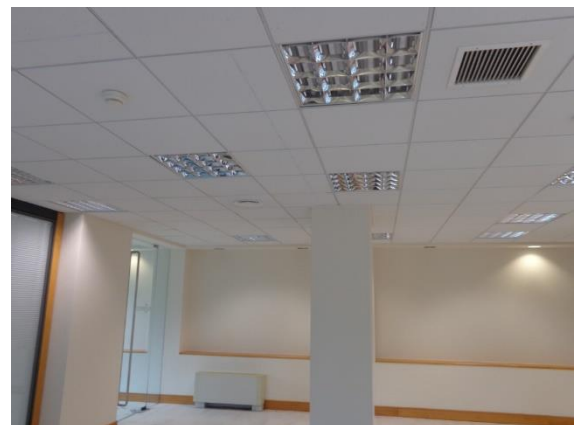
1 st basement vacant office suites
